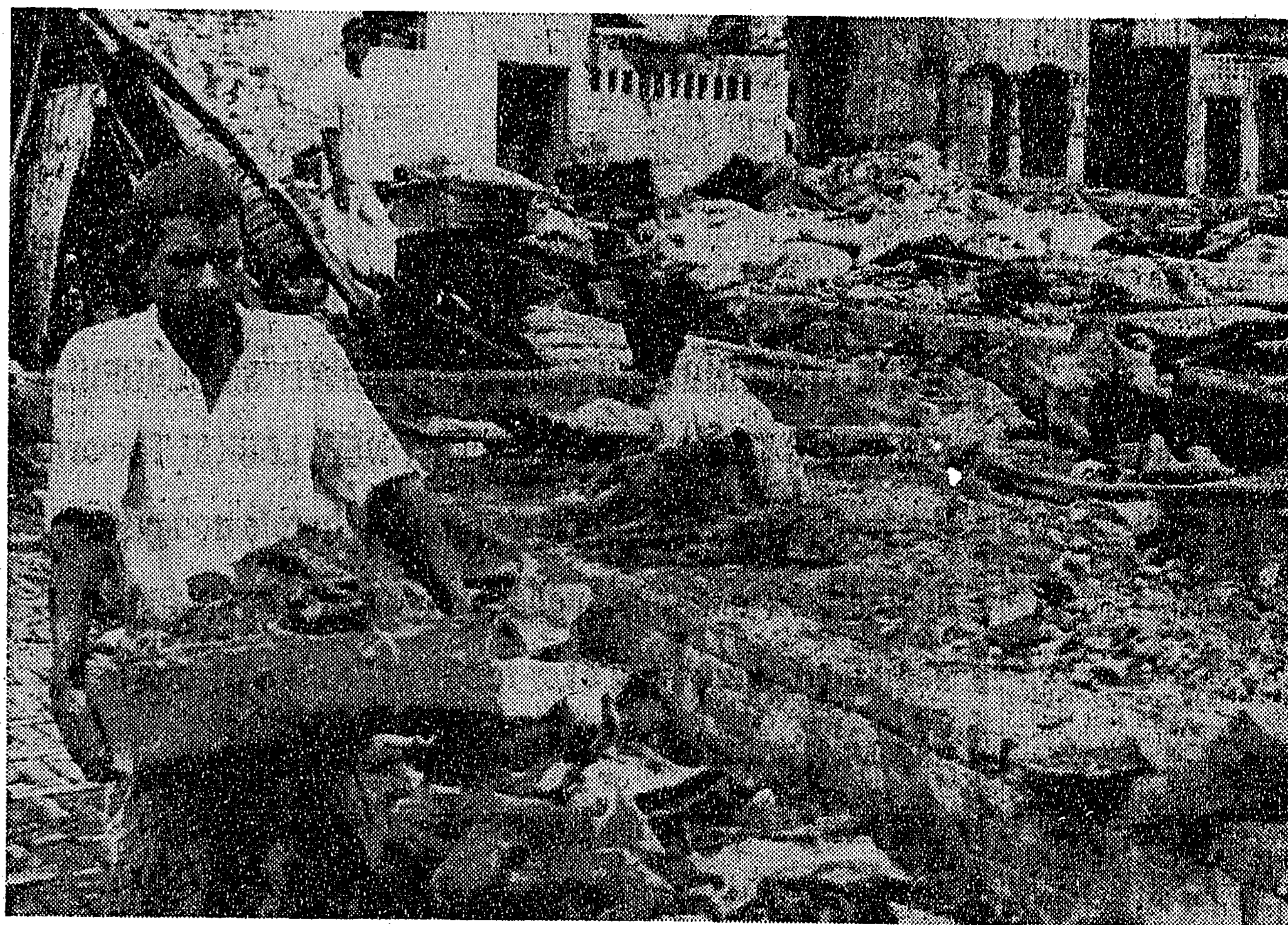
Associated Press AFTER MARKETPLACE WAS BOMBED: Bengalis cleaning up rubble after two-story brick building was shattered in Jessore, East Pakistan, during fighting in May. Bitterness between the Army and many residents persists.
